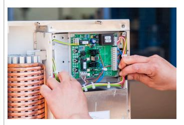
d. Close controller cover and use compressed air to remove dust and dislodge any loose debris
